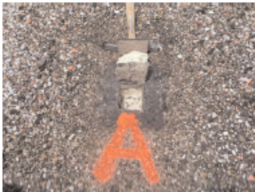
Core Samples Verify the Underlying Construction and Condition
